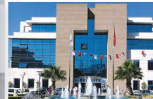
Söke Municipal Building
